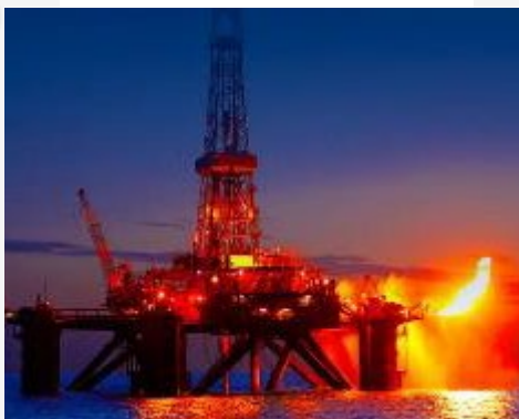
Floating Production Unit
