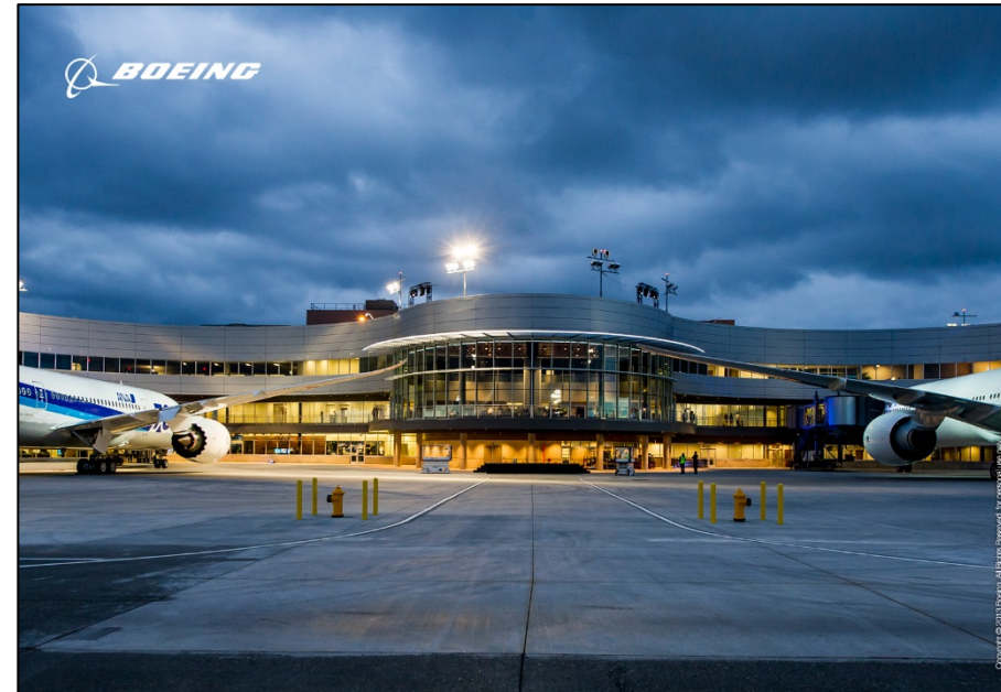
Everett Delivery Center Grand Opening 2013
