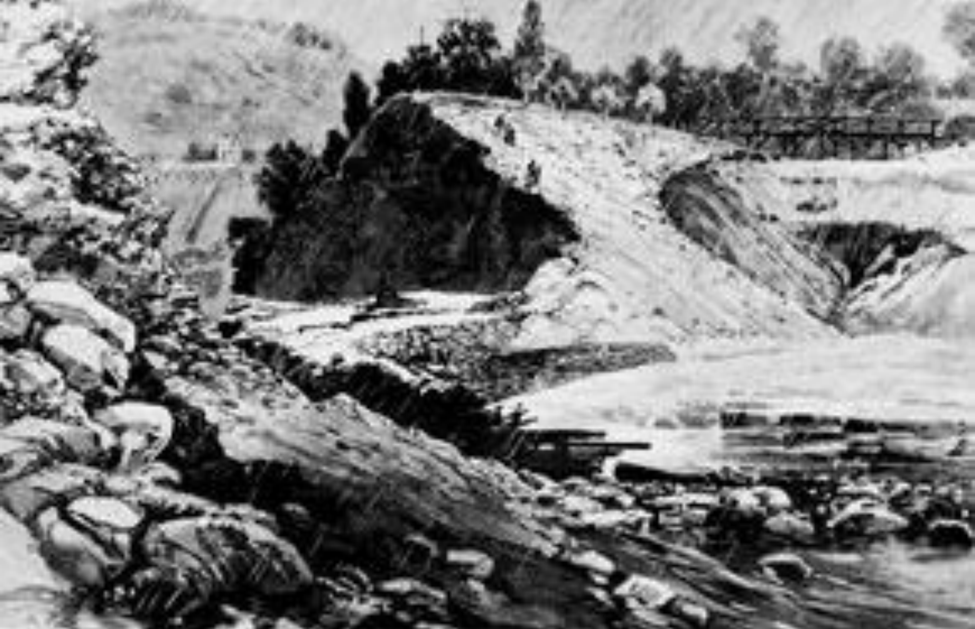
A contemporary illustration of the broken South Fork Dam from Harper's Weekly.
